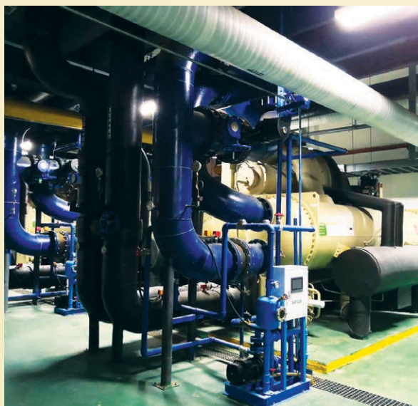
Figure 16: Chiller with Automatic Cleaning System installed
